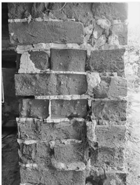
Figure 25. Half-brick cladding on exterior (right) of cheese room, distinctive white mortar in earlier brickwork (left).
