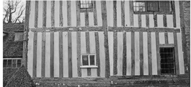
Figure 29. Yelford Manor north wall.
