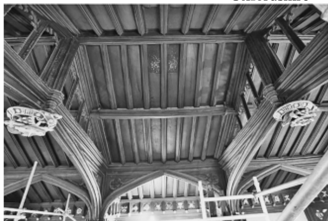
Figure 14. View of the magnificent roof over Wolsey's Great Hall at Christ Church, during urgent repairs in the
