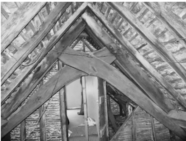
Figure 12. Bay IV, Scissor Brace Truss E, 003.
