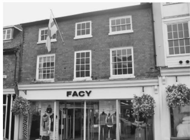
Figure 10. 25 Market Place. North facing c 1800 brick front with three sham windows to create symmetry and hide timber framed structure.
