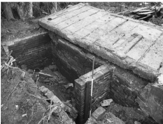
Figure 3. WWII Air raid shelter_Taylors Lane, Lanes End, St Leonards.
