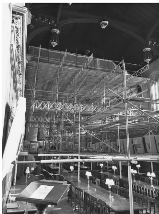
Figure 15. The scaffolding for the roof repairs at the Great Hall, Christ Church, Oxford.
