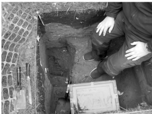
Figure 17. The end of the STGL14 dig as an HV cable is revealed at Terry Stopps' feet
